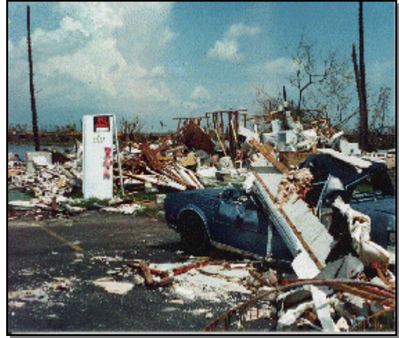
Hurricane Andrew did a lot of damage.
