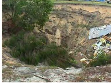
a sinkhole sinkholes
